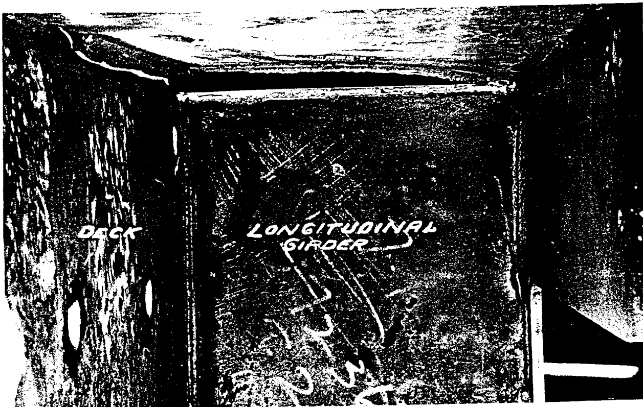
Fig. 40 - Specimen 26: Fracture viewed from below deck, outboard, and fwd. of hatch end beam
