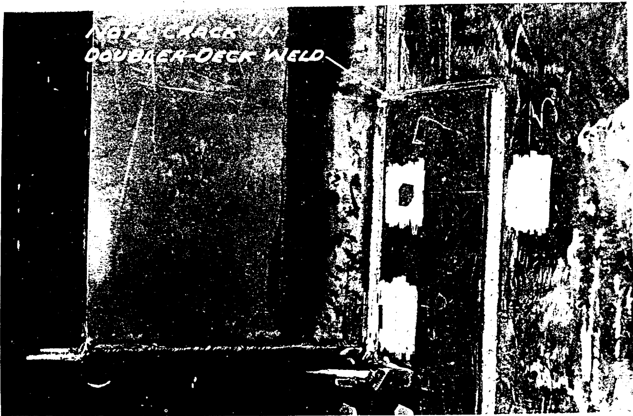
Fig. 31 Specimen 24: Fractures viewed from above deck.
