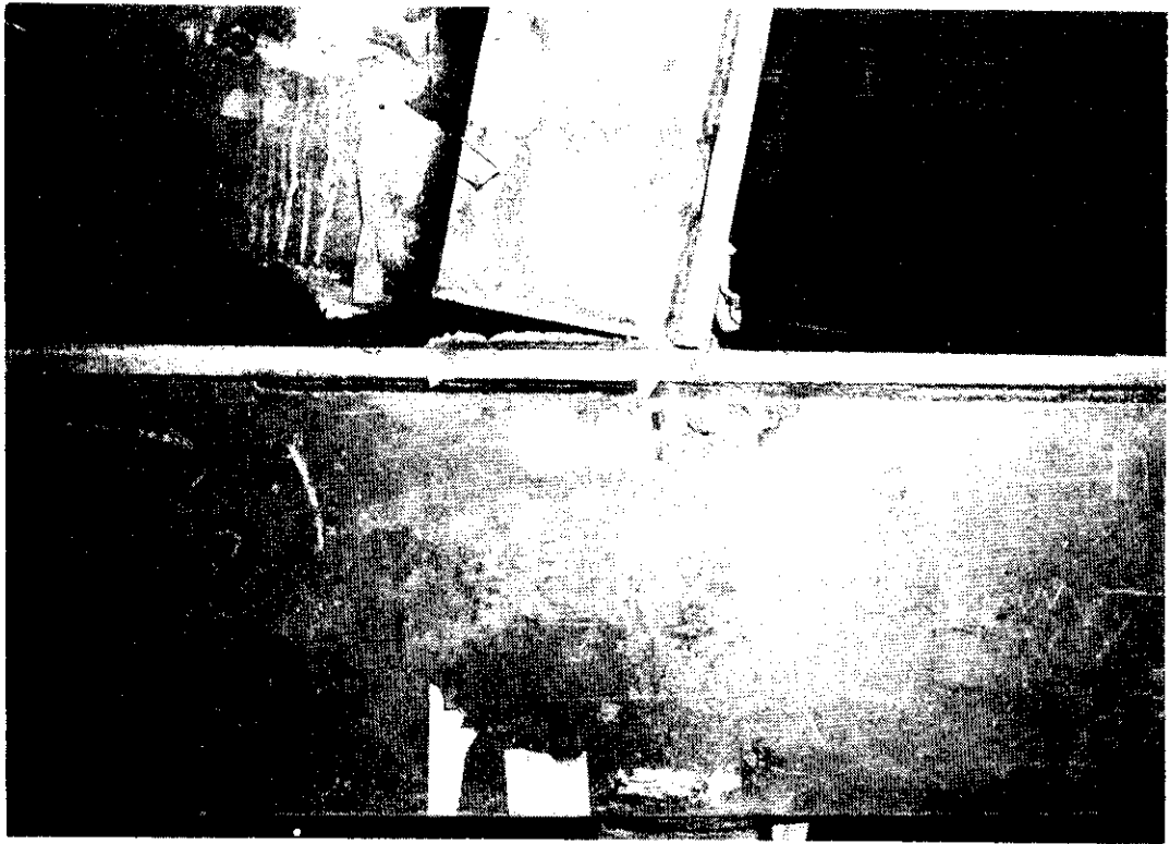
Fig. 17 Specimen 4: View of fracture in weld between longitudinal flange and hatch end beam flange
