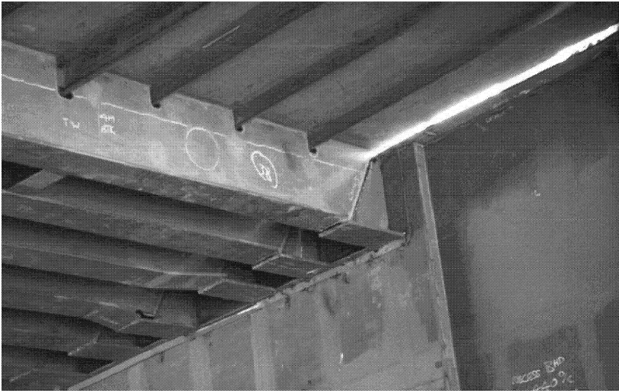
Figure 3 Assembly Work Requiring Overhead Welding
