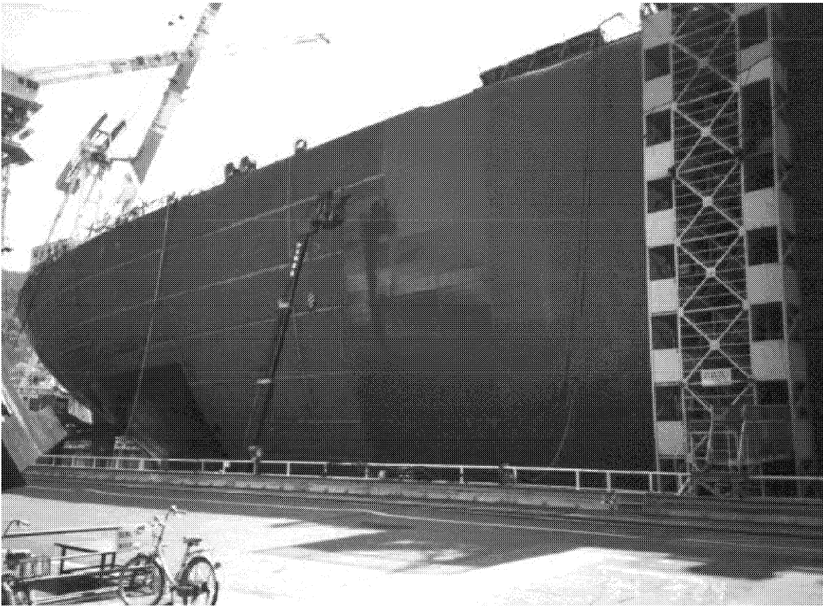
Figure 7 Hull Block Accuracy Improves Painting Productivity and Safety
