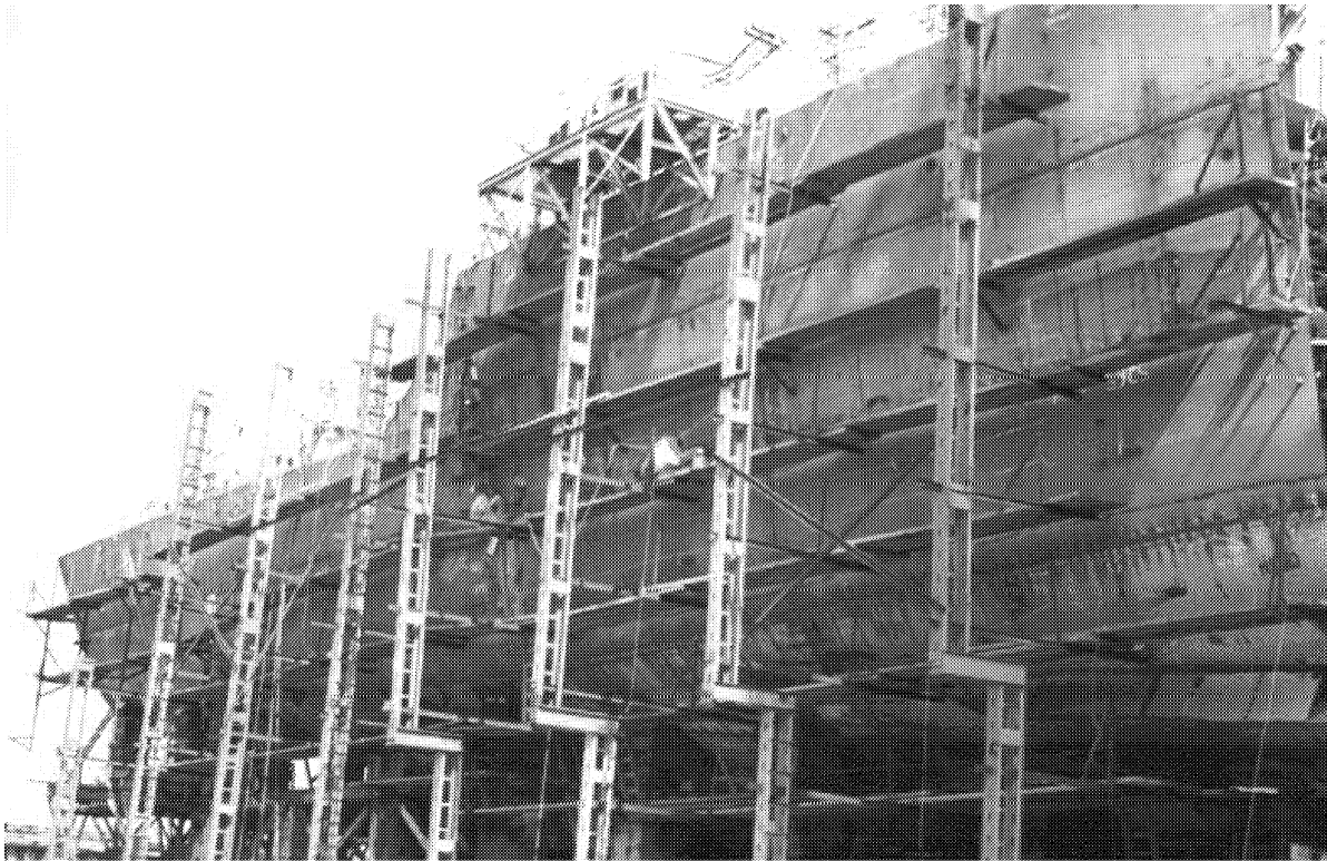
Figure 5 Erection Work, Involving Difficult Fitting and Welding
