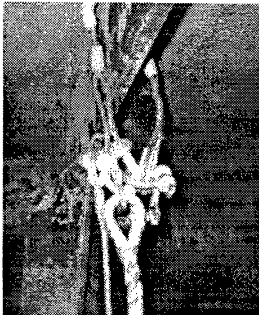
"U" Hook Attached to Underdeck Longitudinal Figure 5-17
