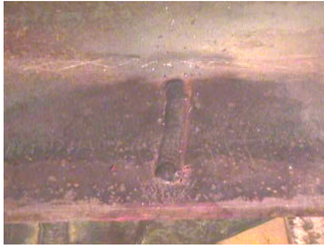
Figure 11-9: Resultant weld between drilled-out crack tips.
