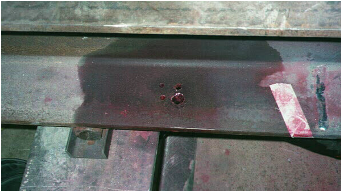
Figure 11-39: Several cracks arrested by hole drilling.
