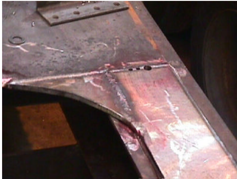
Figure 11-29: Holes drilled to contain crack propagating from internal weld defect.
