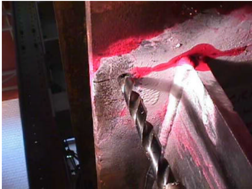
Figure 11-6: Drilling out the crack tips.
