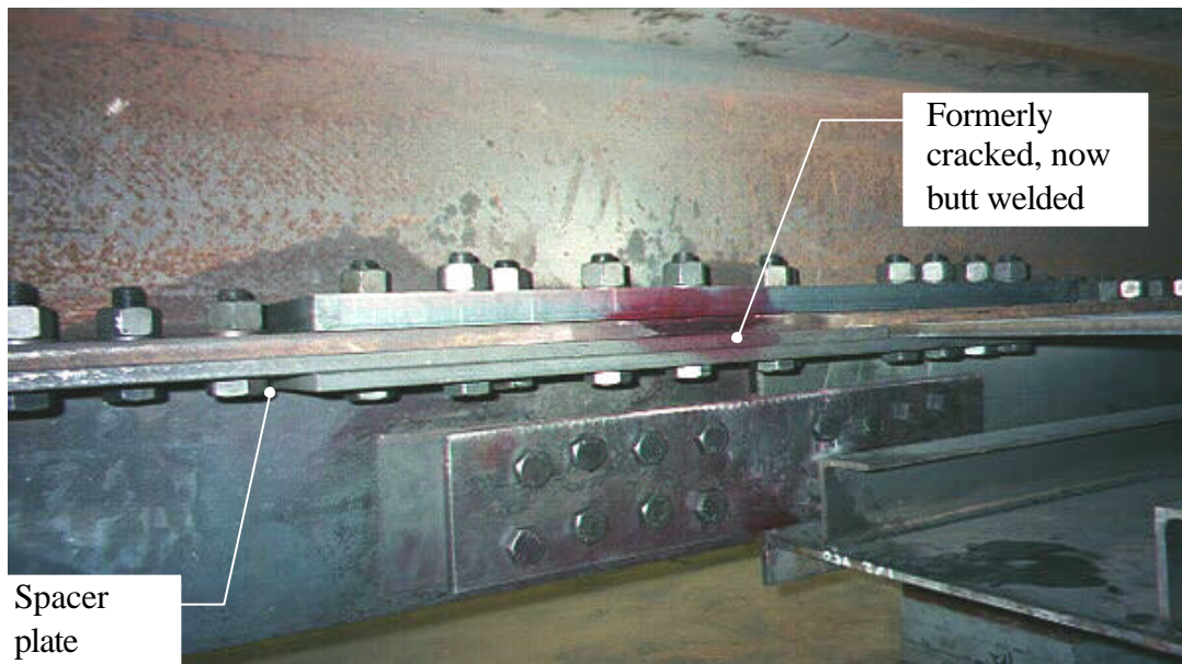
Figure 11-38: Final repair of cracked beam tension flange.
