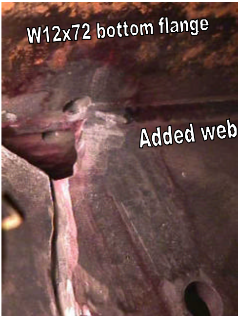
Figure 11-18: Crack faces arc-gouged and crack tips drilled.
