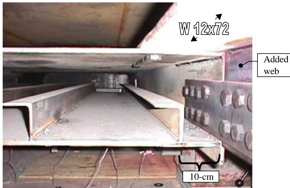
Figure 11-24: Tight clearances for bolting splice plates.
