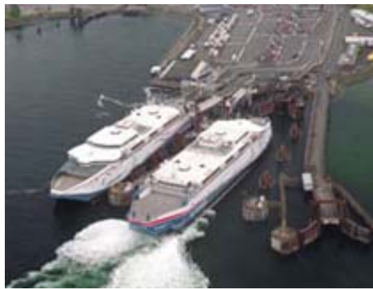
Figure 1: Departure Bay Terminal
