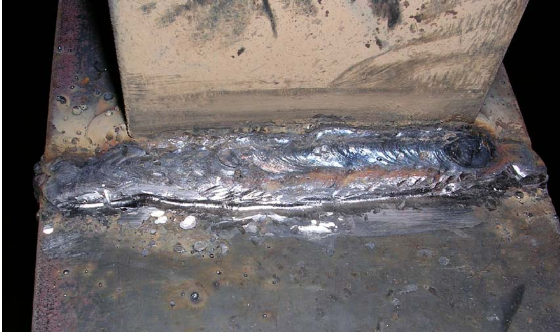
(a) Weld repair of beam flange
