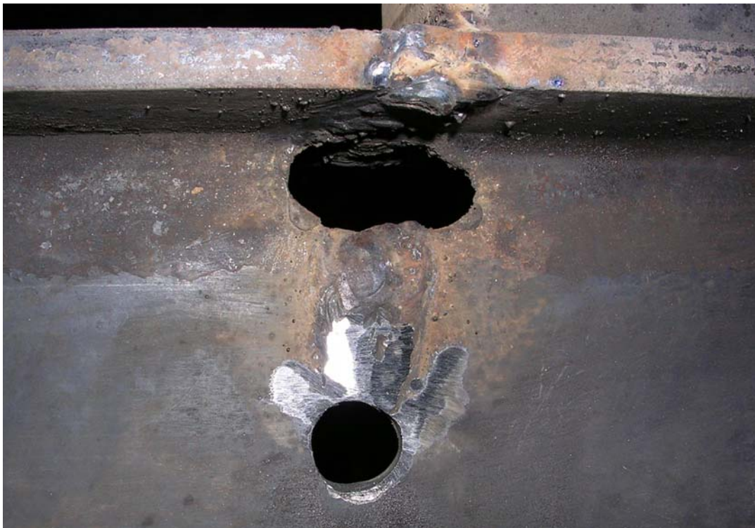
(b) Weld repair of beam web
