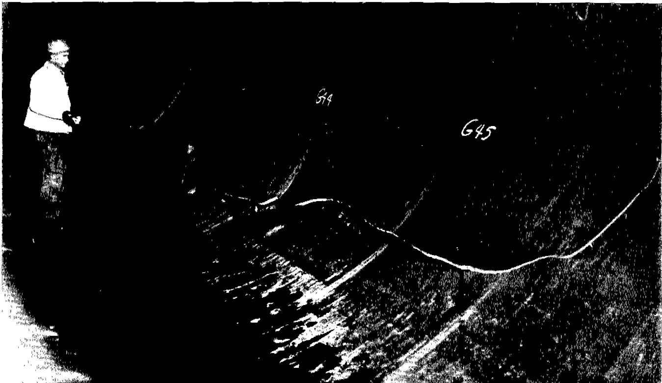
Fig. 30 Penstock failure. Proof hydrostatic pressure test produced a longitudinal brittle failure
