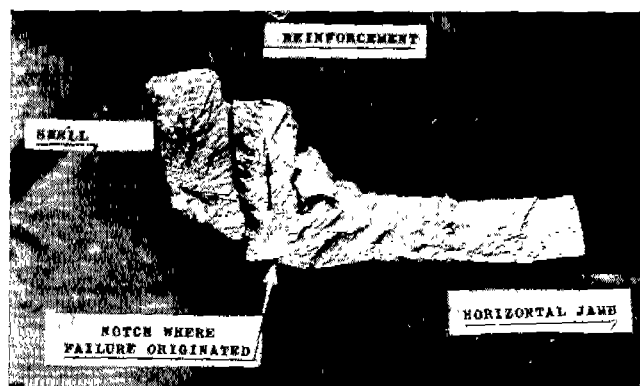
Fig. 18 Origin of fracture in failed crude oil storage tank. Arrow indicates direction of crack propagation
