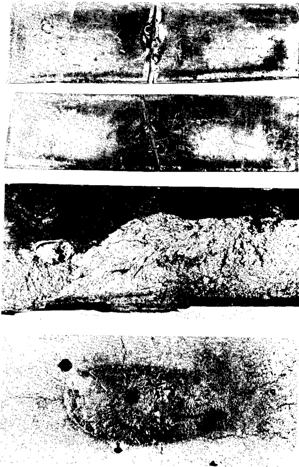
Fig. 8. Top - "A" and "B" Drop Weight Test Pieces with Arc Strike Defects (See Fig. 7) Center - Arc Strike Origin of Fracture in 20" x 20" Weldment. Bottom - Cracks Associated with Arc Strikes; the Crater is Approximately 1/8" x 1/4" actual size.
