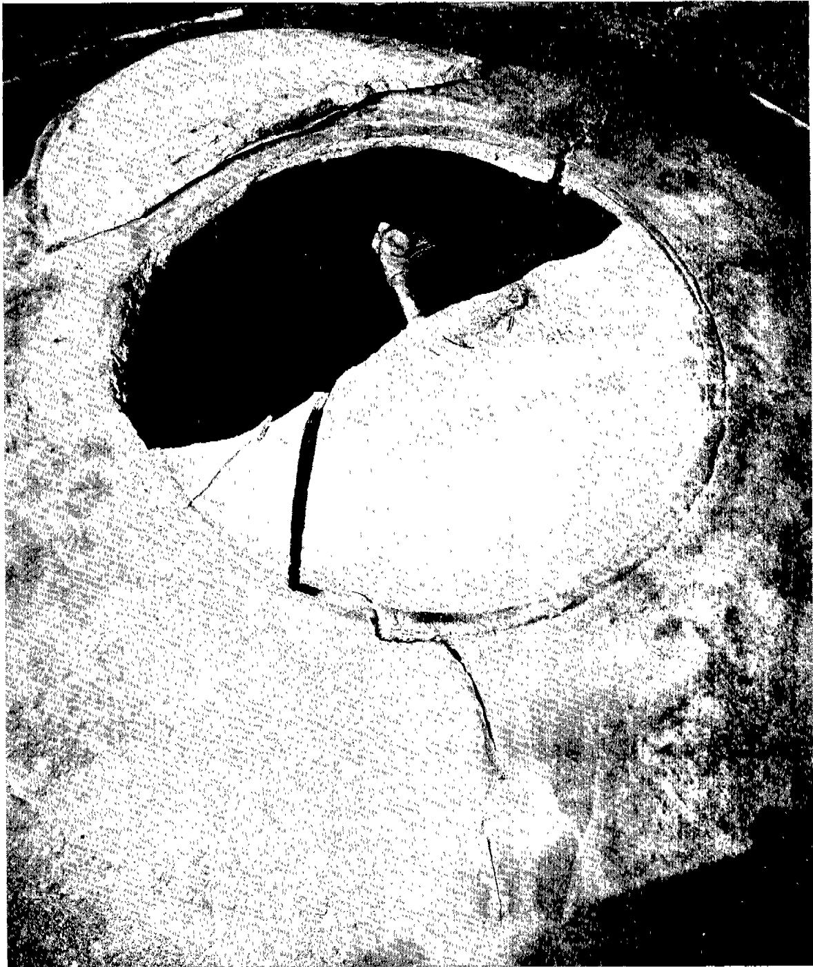
FIGURE D-4. Photograph showing fracture that turned at the E10016 joining weld and followed an old repair weld. It finally stopped in unrepaired T-1 after propagating 15-1/2 in. into the sphere on one side and 12 in. on the other.
